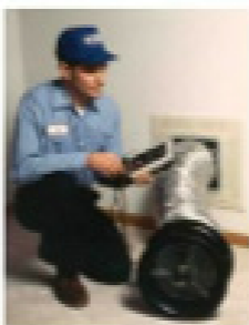
Photo of Man Conducting Duct Blaster Test: A duct blaster test evaluates the leakiness of the duct system.
